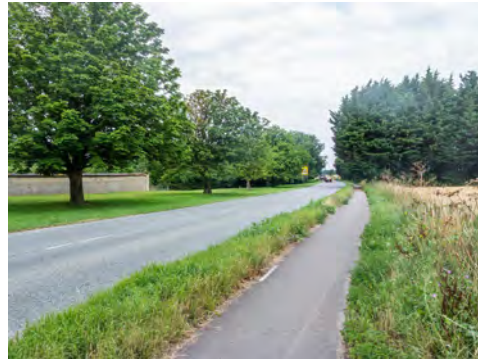
Image 9: Village Gateway 1 - West (B1102) looking out of the village towards Lode
